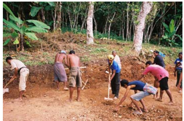
Farmers preparing a concrete slab for coffee processing.
